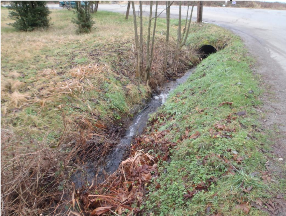
Photo 2: Soule Creek on 2661 F-G Rd and culvert to estuary
