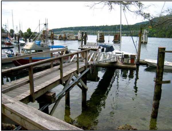
Figure 4: Existing pier and ramp
