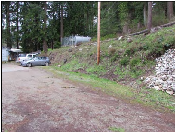
Figure 6: Parking area looking west
