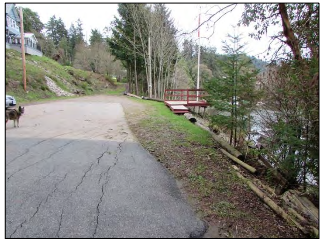
Figure 7: Parking area looking east
