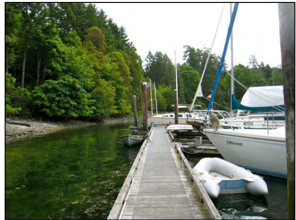
Figure 5: Portion of existing dock
