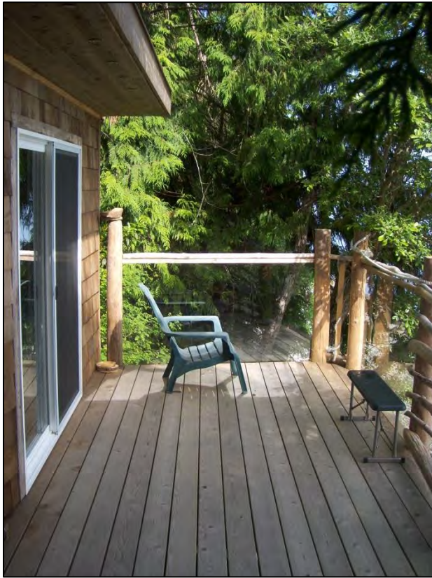
Figure 5: Deck adjoining accessory building.
