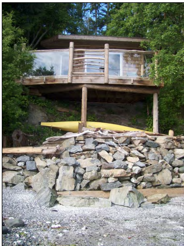
Figure 3: View of rip-rap and structure from shore
