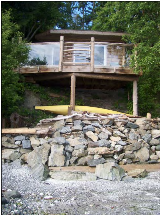
Figure 3: View of rip rap and structure from shore
