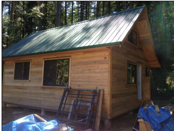
Figure 3: Exterior of subject building at time of site visit.
