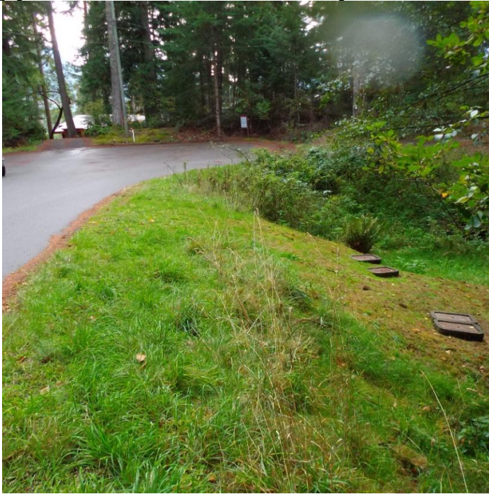
Photo 5: Looking down W side road shoulder over water boxes, proposed route for water pipeline. Grassed ditch reach 2 enters picture from center right to culvert at center.
