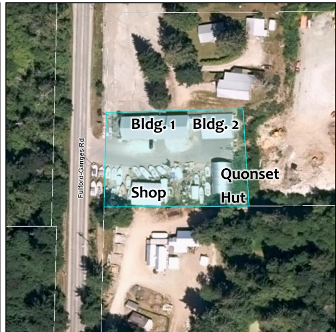
Figure 2: 2013 Orthophoto of Subject Property
