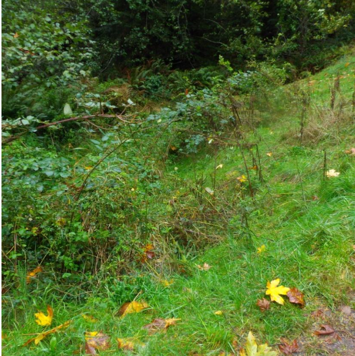
Photo 3: From culvert looking up ditch reach 2.
