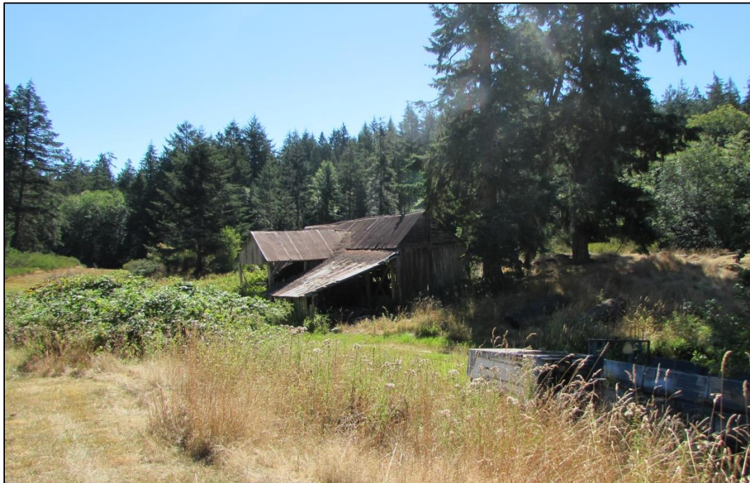
Figure 4: Historic farm buildings on proposed Lot B.
