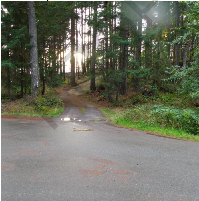
Photo 6: Culvert under culdesac lower right. Buried water pipe will follow shoulder up to new driveway in center.
