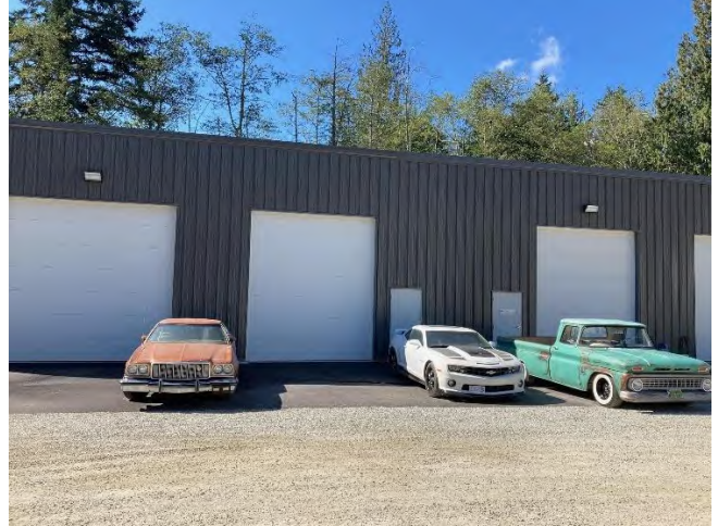
EXISTING STORAGE BUILDING #1
