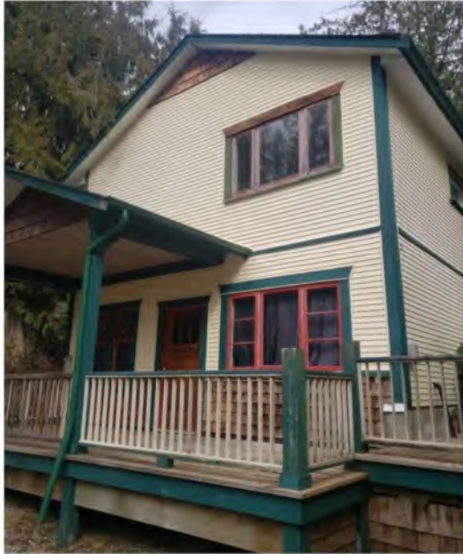
South Elevation View
