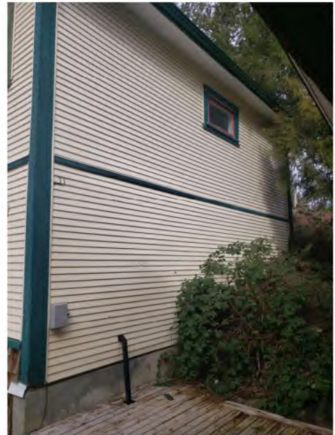
East Elevation View
