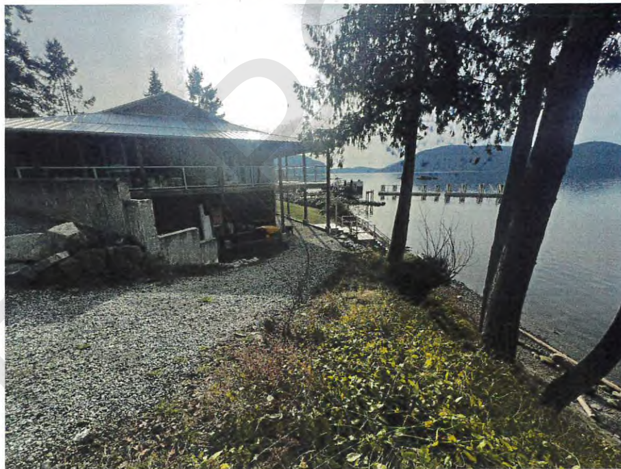
2. View southeast toward existing building
