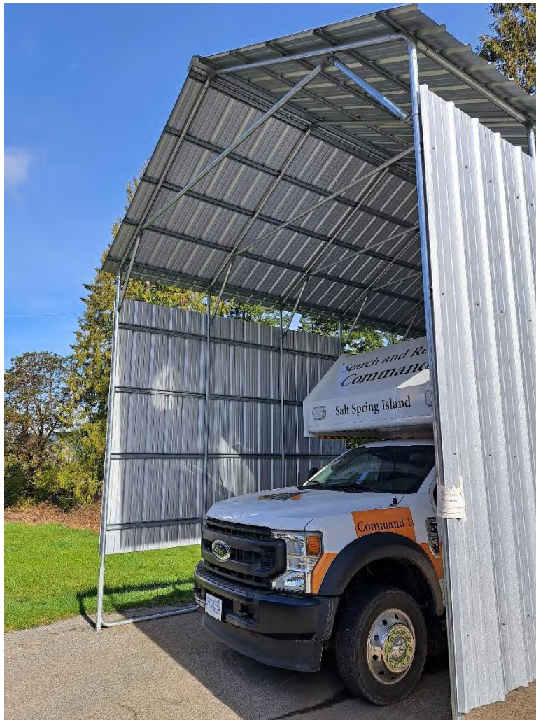
Existing structure, front view
