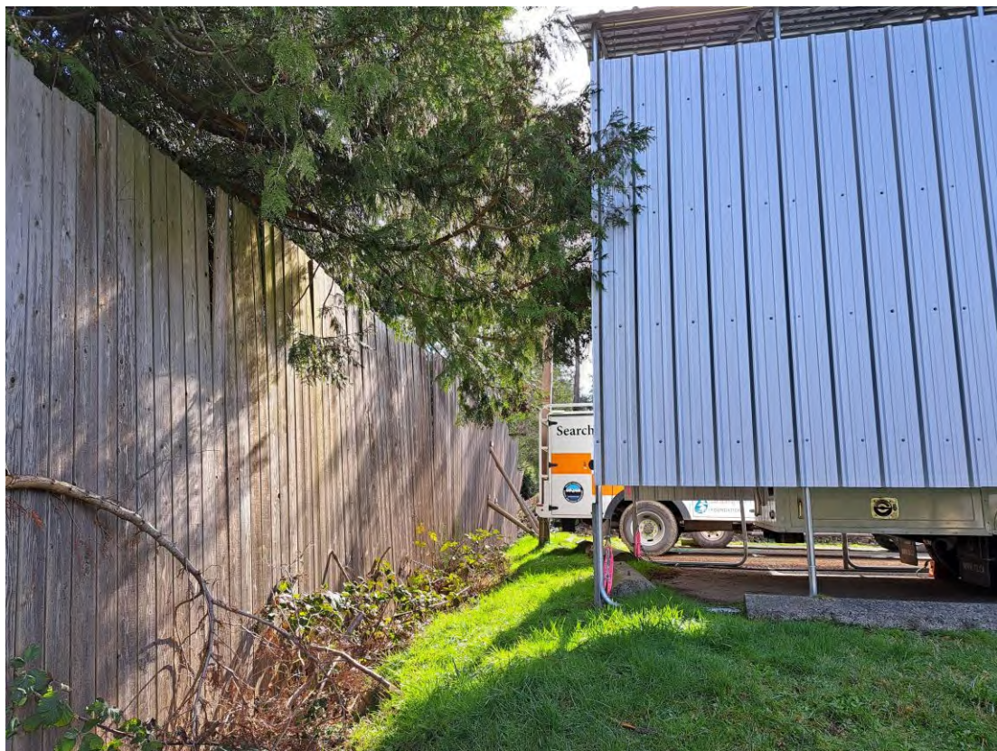
Existing structure in rear lot setback, looking south
