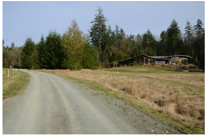
Driveway and Single-Family Dwelling on Subject Property
