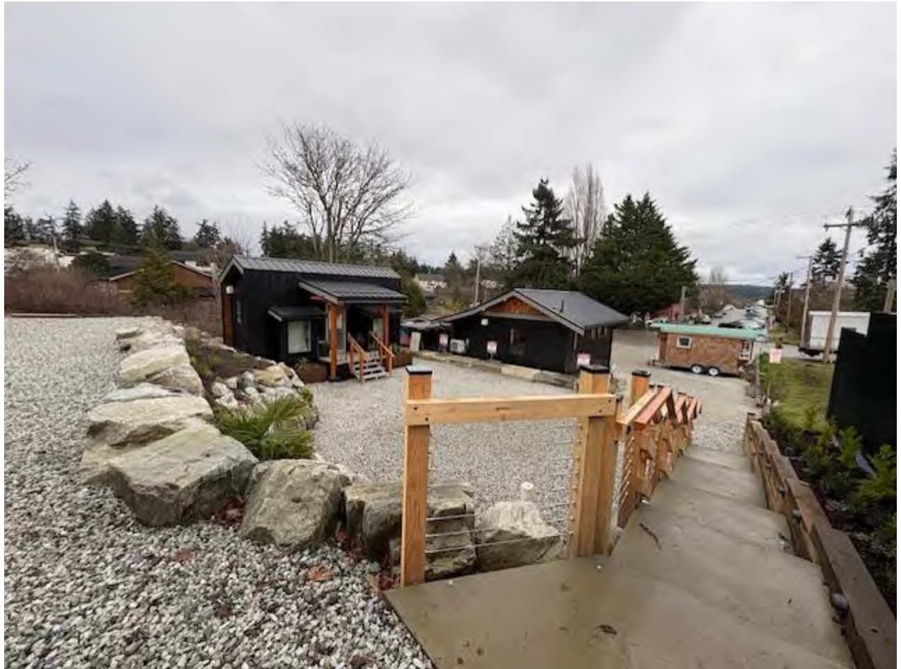
Figure 9 – View to the North East
