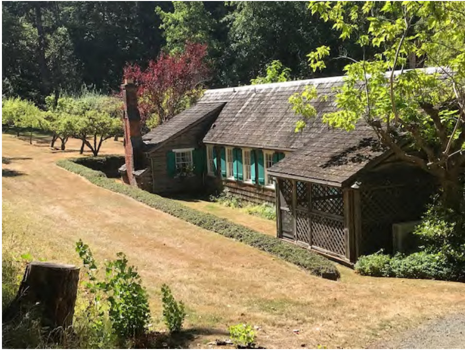
Fig. 3. East side Menschel Residence. Note excavated area for original existing structure. Small modular additions will be made to the south side (orchard side) of the existing structure.
