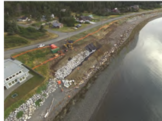
Pictures 3 and 4 depict Low Bank Beaches in Comox, B.C. Rocks and logs are used as a natural approach to slow tidal flows and to prevent erosion.
