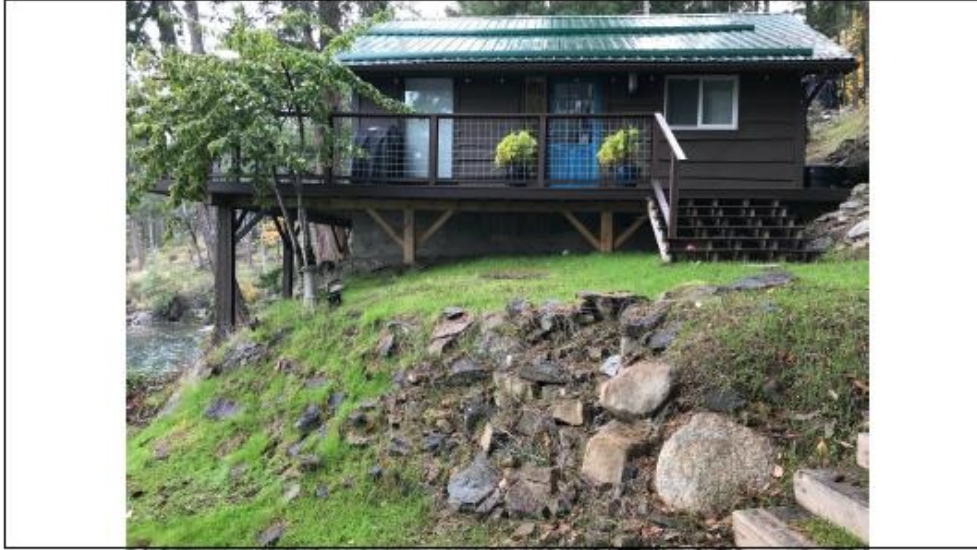
South side of existing house looking north. Proposed entry would be placed in between the two windows
