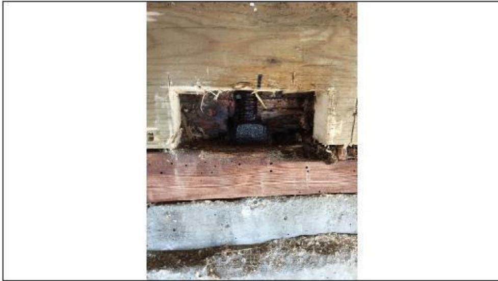
Old square-headed bolts used to connect framing to foundation.
