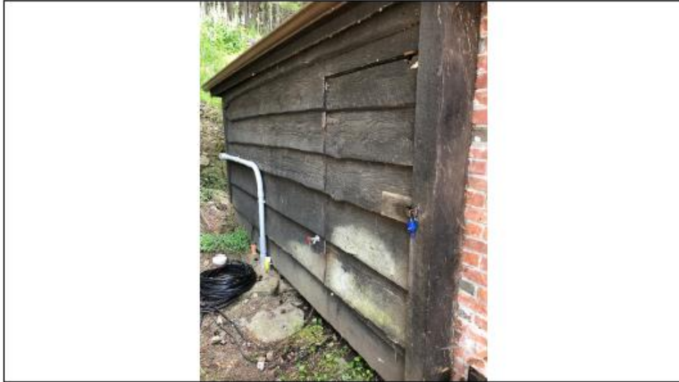
1" thick wide-plank cedar siding.
