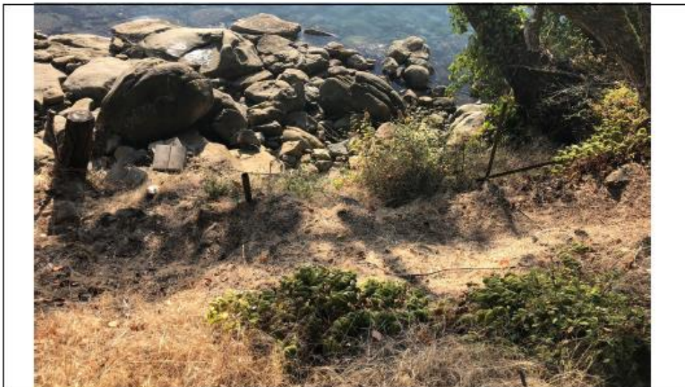
Looking west down at foreshore area from shoulder of slope.
