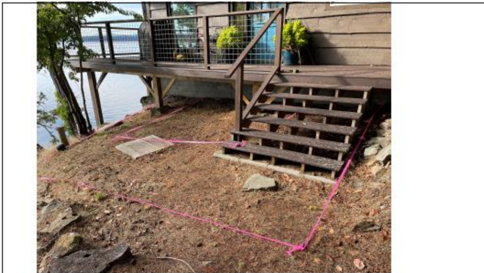
Close up photo of location of proposed new entry. Pink ribbon denotes approximate outer limits of addition and deck.
