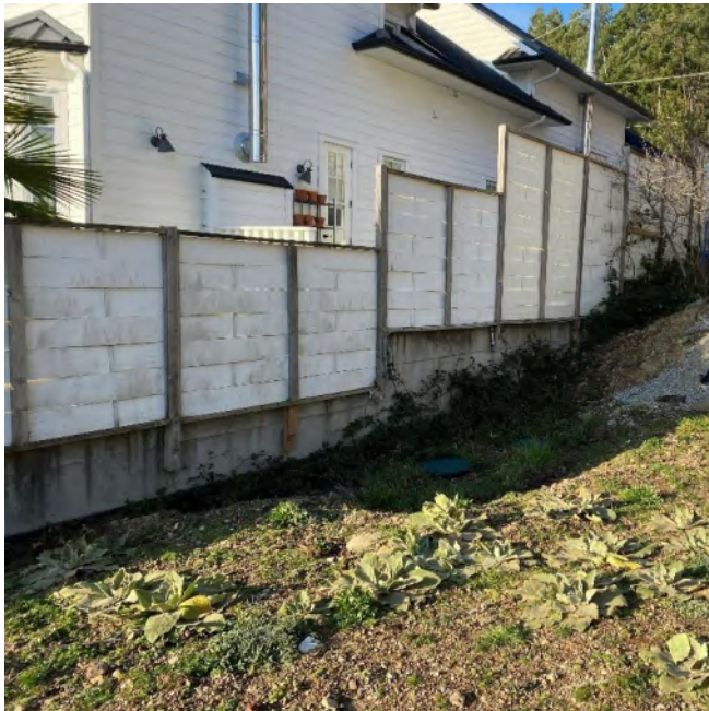
West Interior Side Lot Line and Neighbouring Lot/Dwelling
