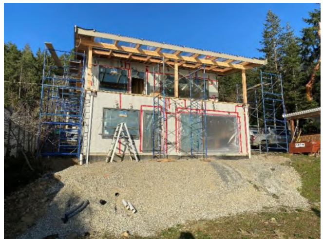
Single-Family Dwelling Under Construction
