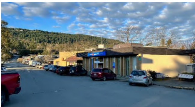
Subject building and existing signage from Fulford-Ganges Road
