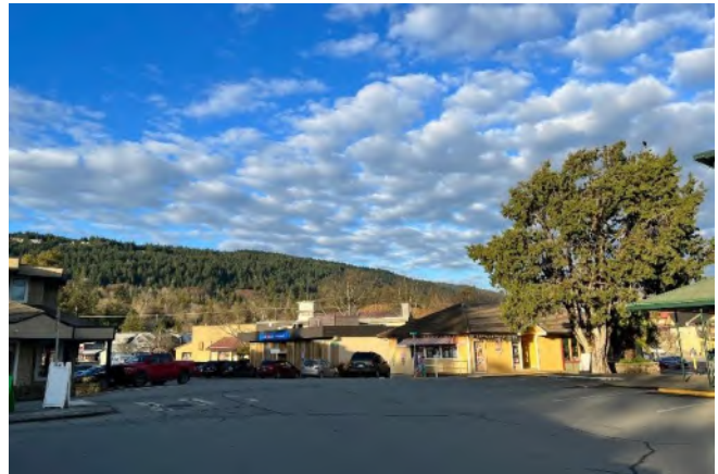
Subject building and existing signage from Fulford-Ganges Road
