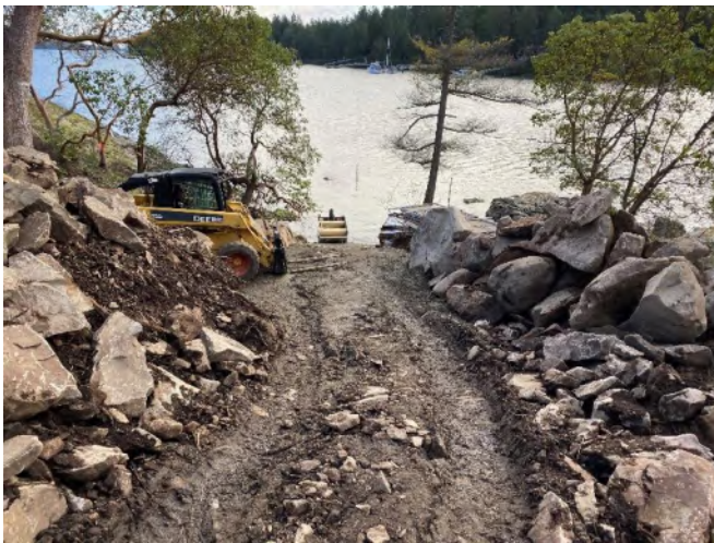
Photo 3: Islet access point. Retaining wall elements visible.
