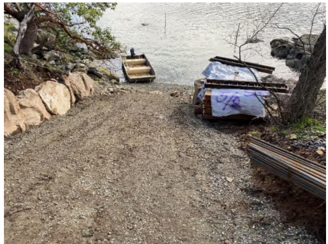
Photo 4: Islet access point. Retaining wall elements on left side. Soil/fill deposit evident in foreground.
