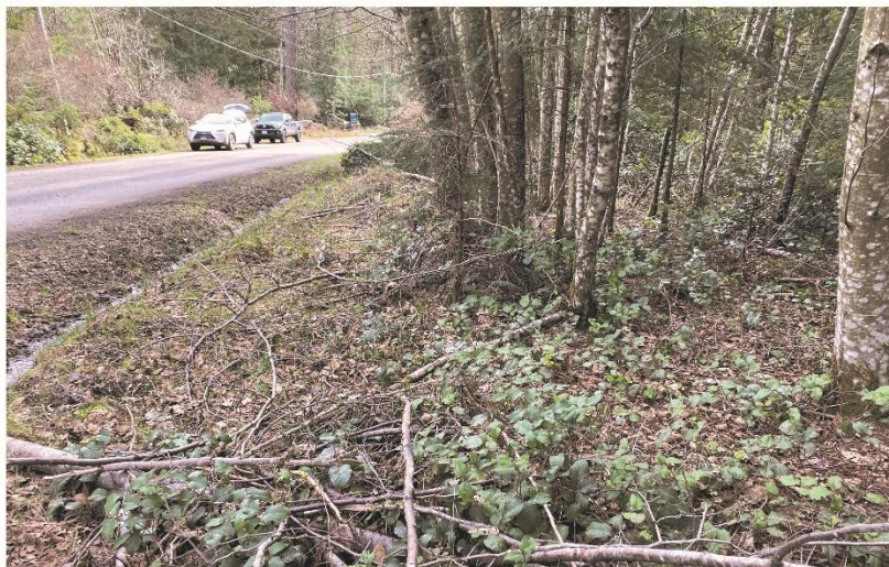
Upper drainage ditch (Reach 1 -View southeast along Meyer Rd.)
