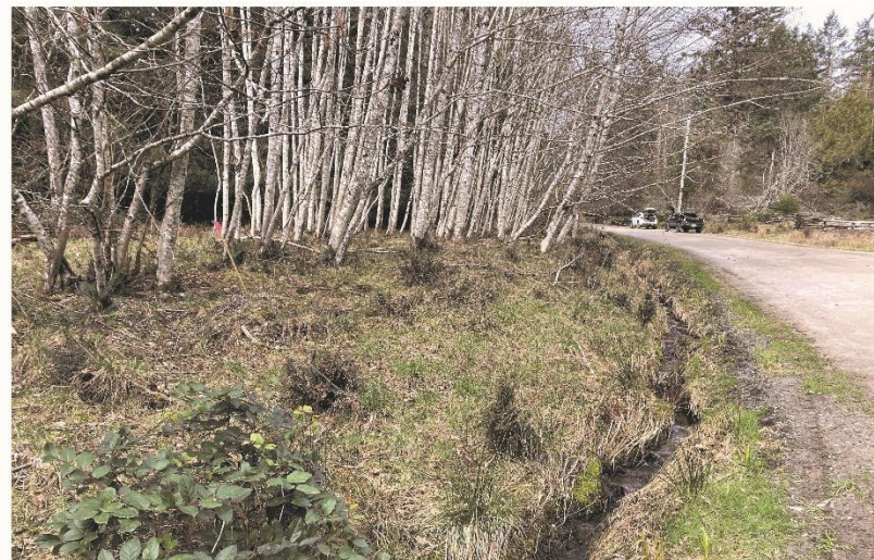
Lower Watercourse (Reach 2 -View northwest along Meyer Rd.)
