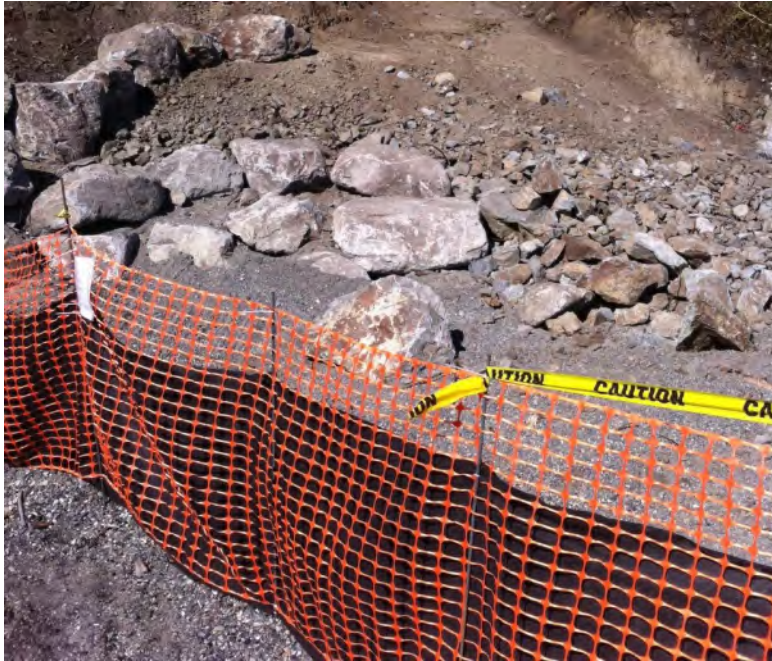
Photo 3. Example erosion control to protect marine environment during work.
