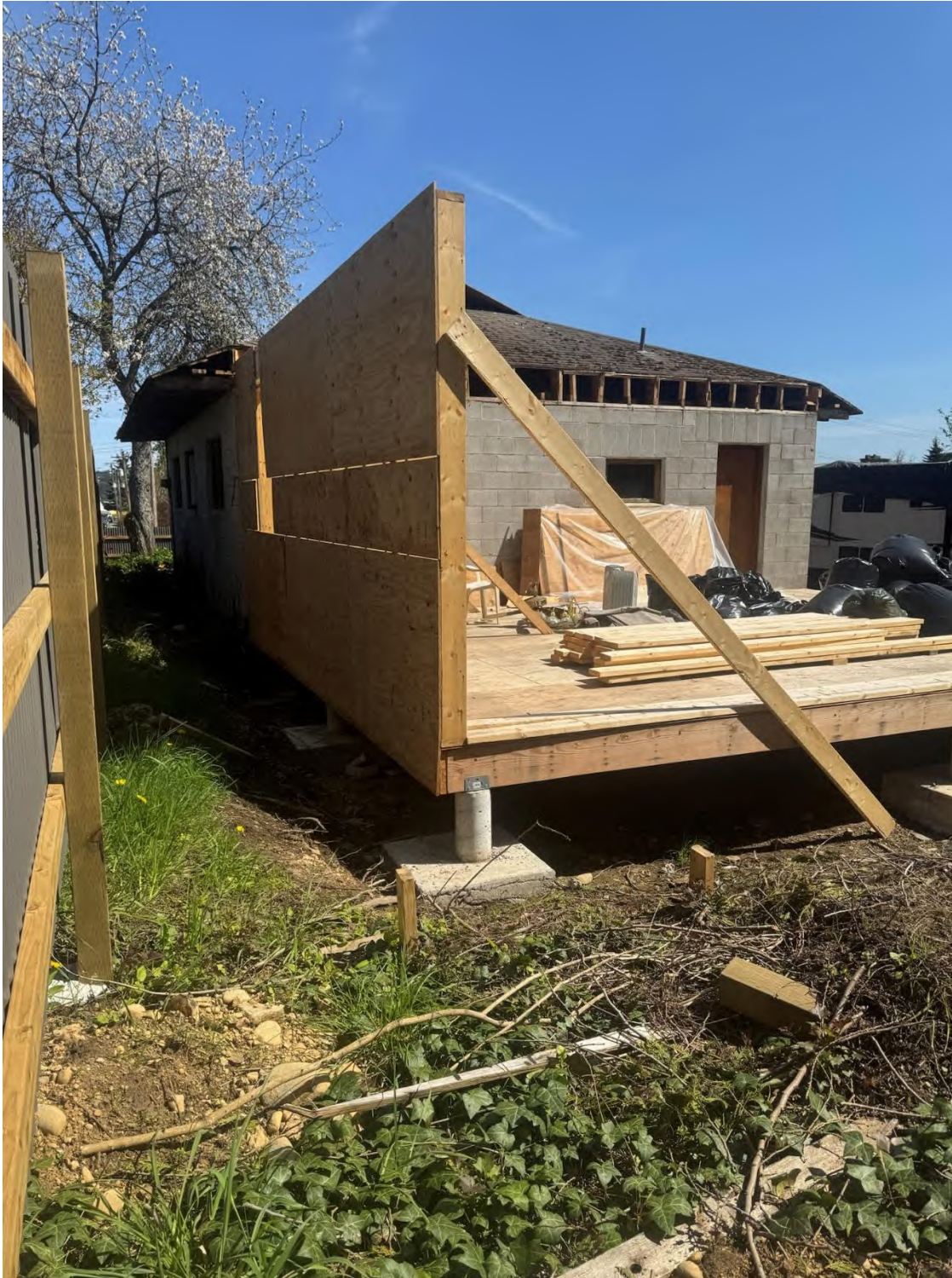
Figure 9 – View from the North-West
