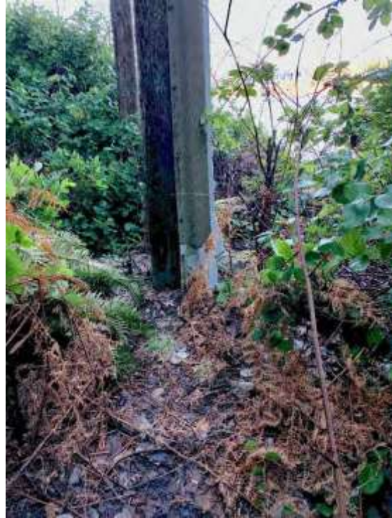
Photo Point 8. South side of BC Hydro pole. Photo: C. Schaefer.
