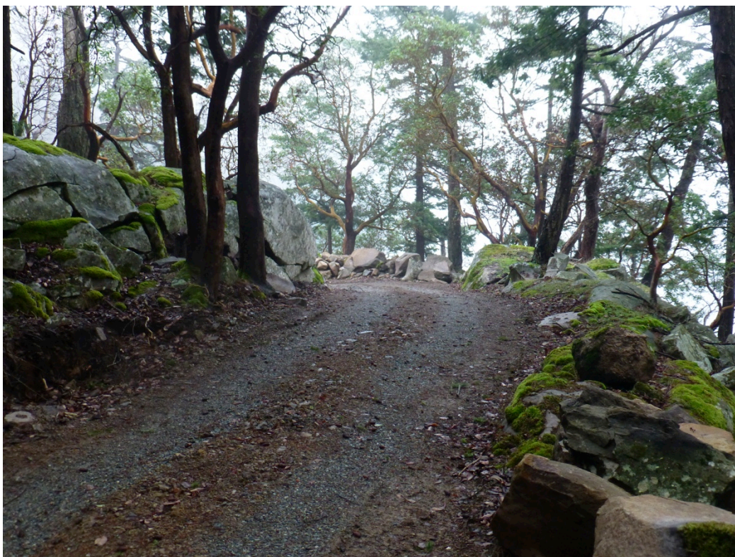
Figure 7. The first leg of new driveway. Photograph taken, January 10, 2015.
