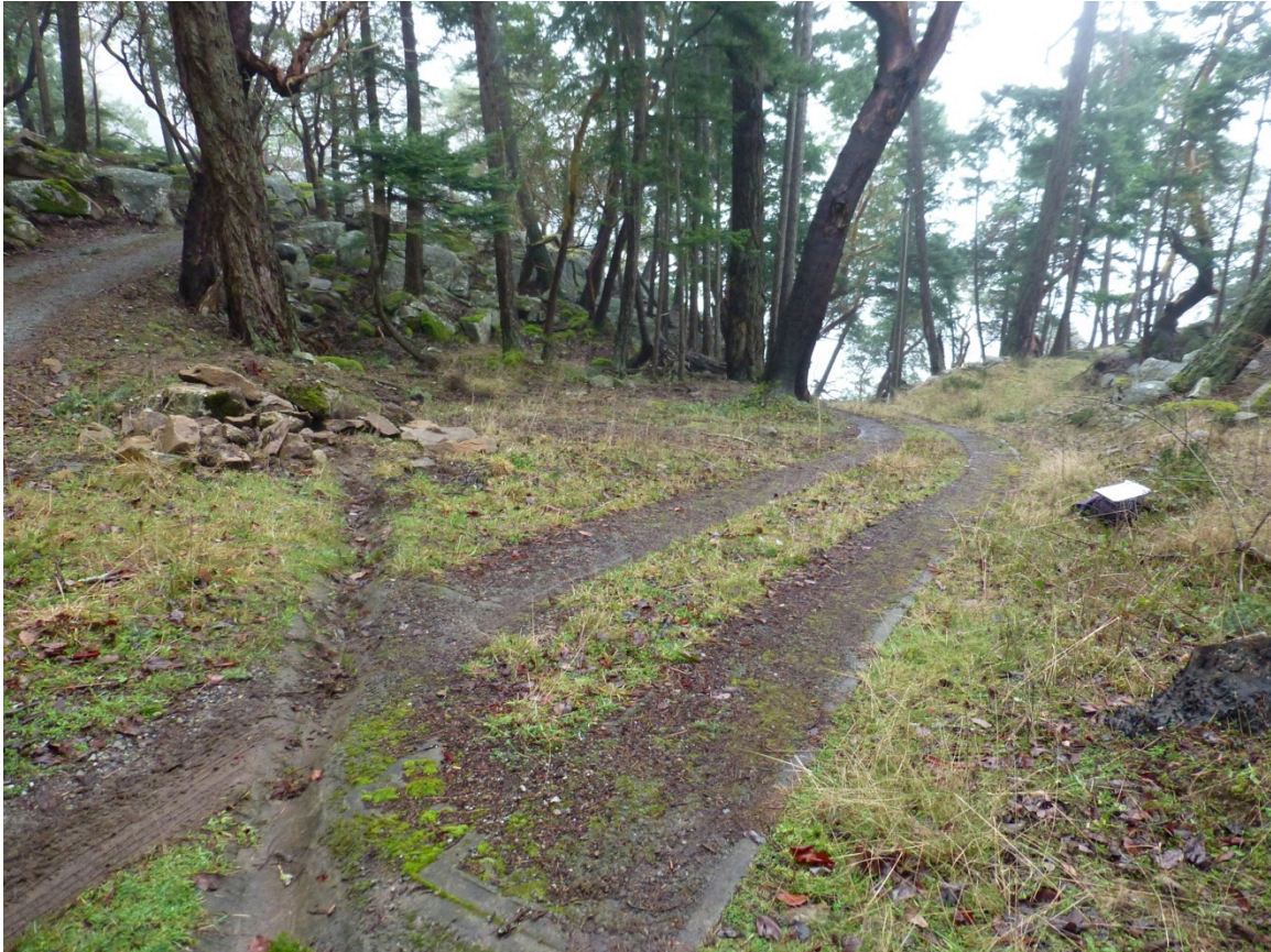
Figure 9. View of the upper portion of existing driveway (upper section of new driveway is seen in upper left corner of photo. During reclamation cement slabs should be removed and native tree species re-established along its entire length. A deer/goat exclosure plot would work well here. Photo taken, January 10, 2015.
