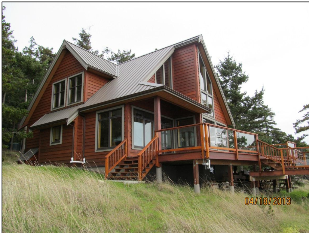
Picture 1: Looking northeast towards dwelling unit
