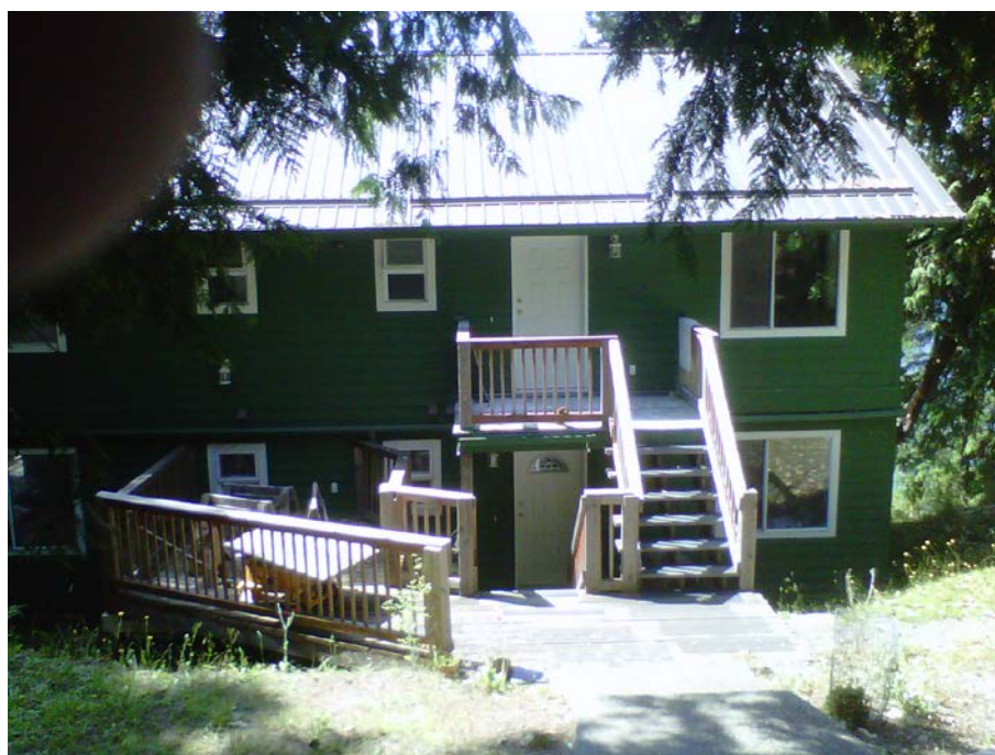
Photo 1 – Front of residence
