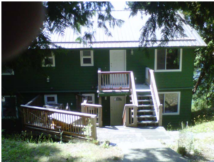
Photo 1 – Front of residence
