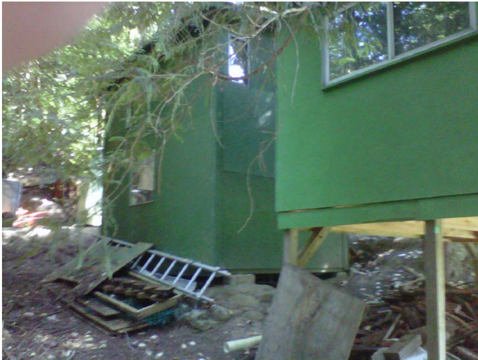
Photo 3 – Buildings A and B
