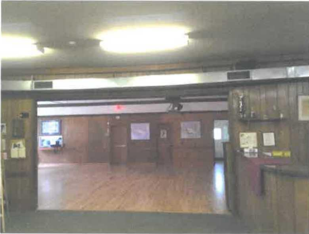
Hall to Lounge beam to be rebuilt and ducts hidden
