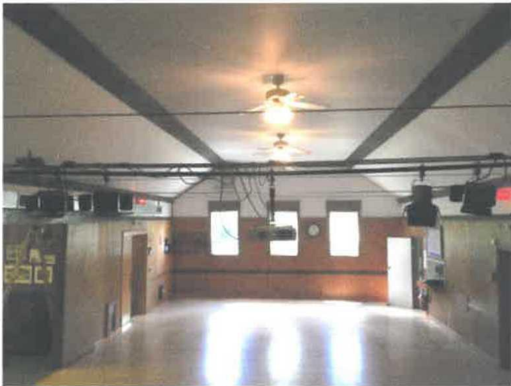
View from Stage -new lighting truss will raise lights to proper ceiling position
