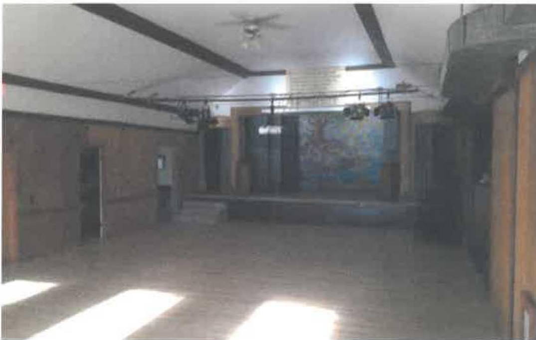
Hall- ducts on right and wash room entrances removed, new lighting truss,
