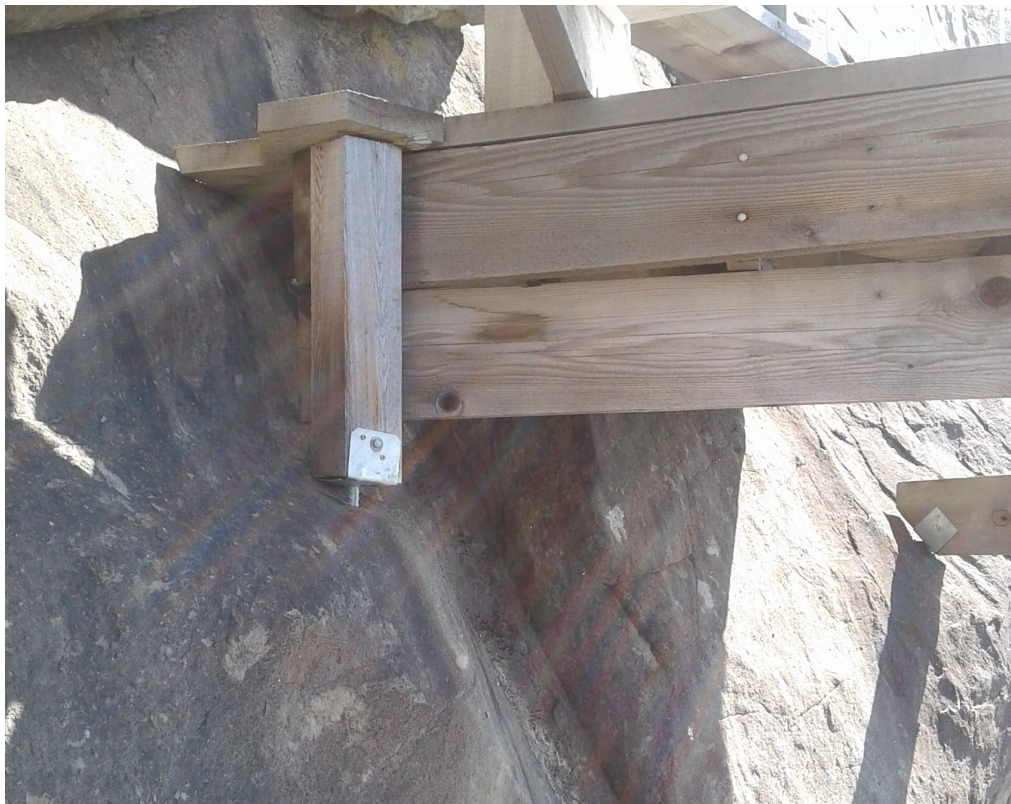
Plate 7b. Galvanized rebar saddle brackets supporting stairs at 130 Cliffside Rd., Saturna Island BC.
