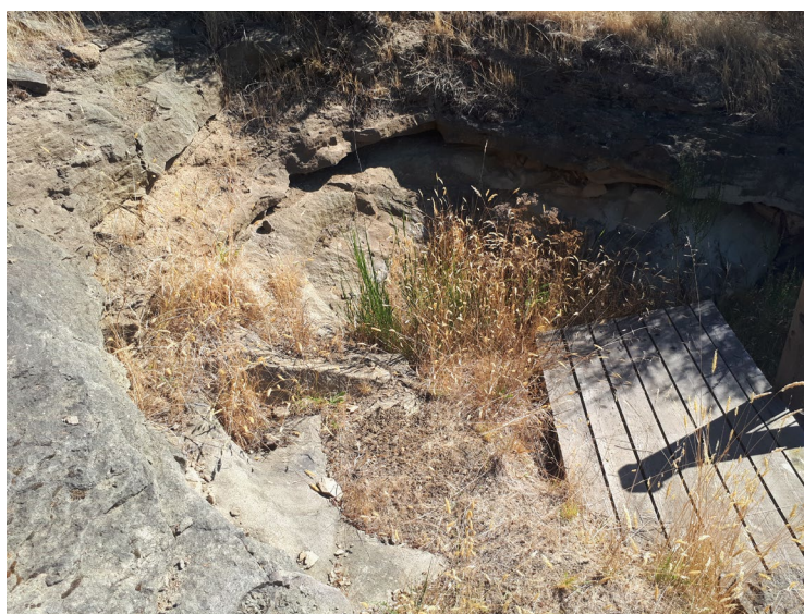
Plate 1. Alcove created by historical blasting work at the top of the cliff, forming the present top landing of the stairs at 130 Cliffside Rd., Saturna Island BC.
