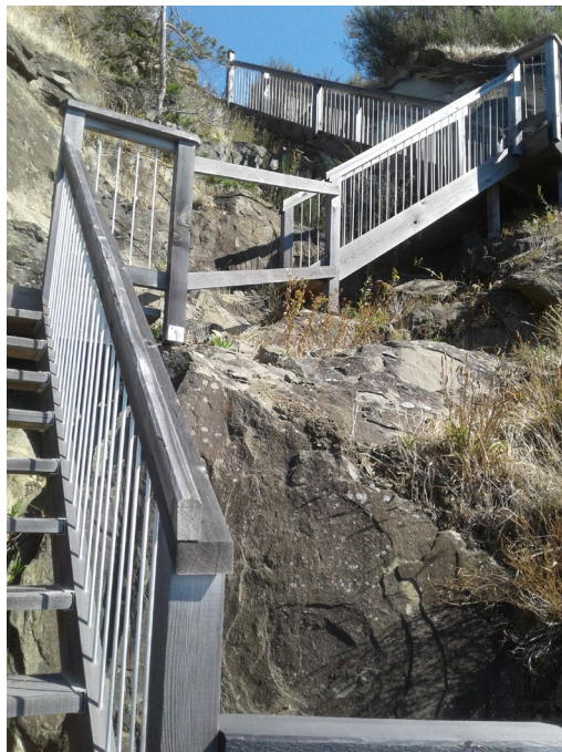
Plate 6. Overview of rockface where stairs have been built at 130 Cliffside Rd., Saturna Island BC.
