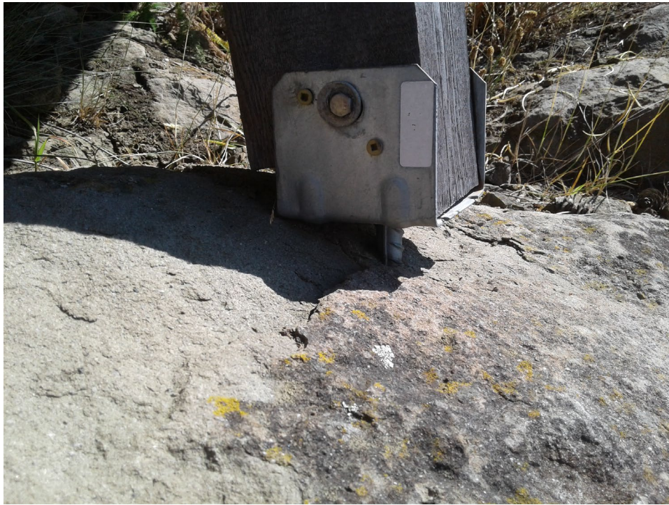
Plate 7b. Galvanized rebar saddle brackets supporting stairs at 130 Cliffside Rd., Saturna Island BC.
