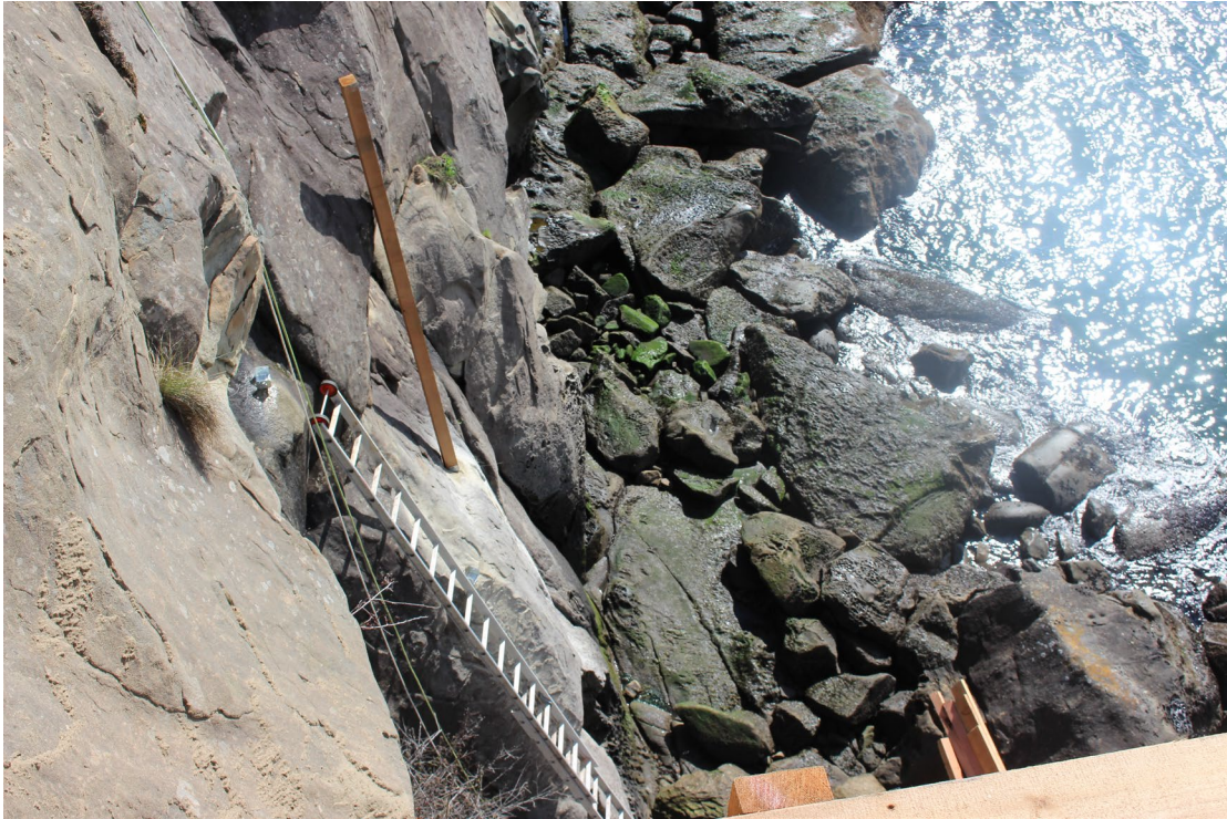
Plate 11. Installation of wooden stairway on rock face in Bluffs Ecosystem DPA at 130 Cliffside Rd., Saturna Island BC. (Photo courtesy of Glenn Fjordbotten)
