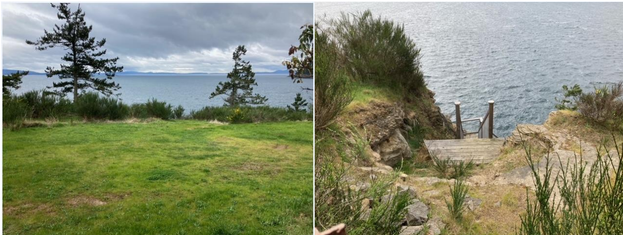
Figure 4. Site photos showing significant land clearing in DPA 2 and blasting of opening on cliff edge
