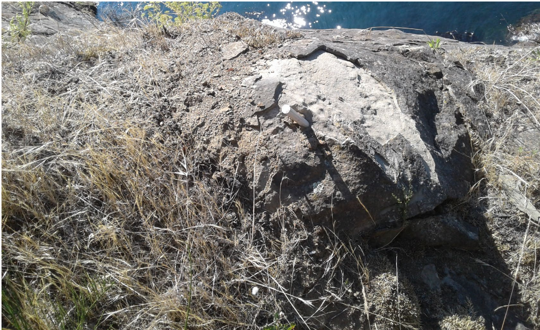
Plate 8. Removal of soil veneer and associated vegetation on rock bluff resulting from stairway construction in the Bluffs Ecosystem DPA at 130 Cliffside Rd., Saturna Island BC.
