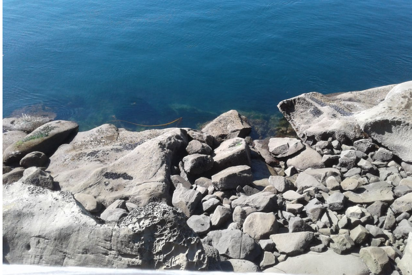
Plate 5. Large rock debris at base of stairs showing evidence of previous rock removal by blasting at 130 Cliffside Rd., Saturna Island BC.
