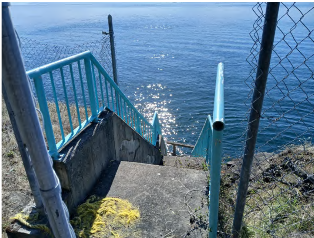
Plate 2. Small man-made depression with local sandstone and concrete pieces at 180 & 182 Cliffside Road, Saturna Island BC.
