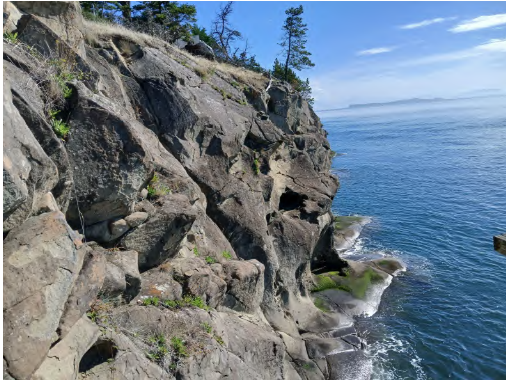
Plate 7. Evidence of seasonal shoreline erosion due to wave action at 180 & 182 Cliffside Road, Saturna Island BC.
