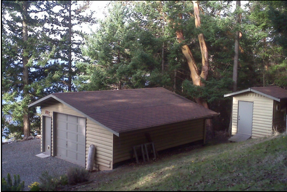
Photograph 2: Existing Accessory Buildings (garage and shed)
