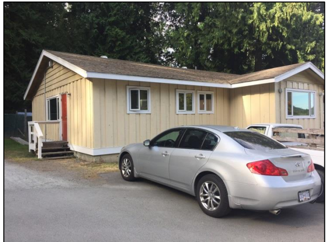
Image 8: However, the applicant sent a subsequent image demonstrating that the administration building has been repainted.
