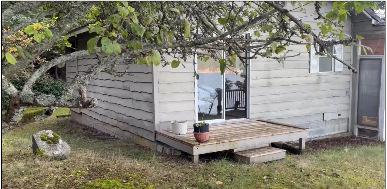
EXISTING PORTION OF DWELLING TO BE REPLACED, LOOKING WEST
