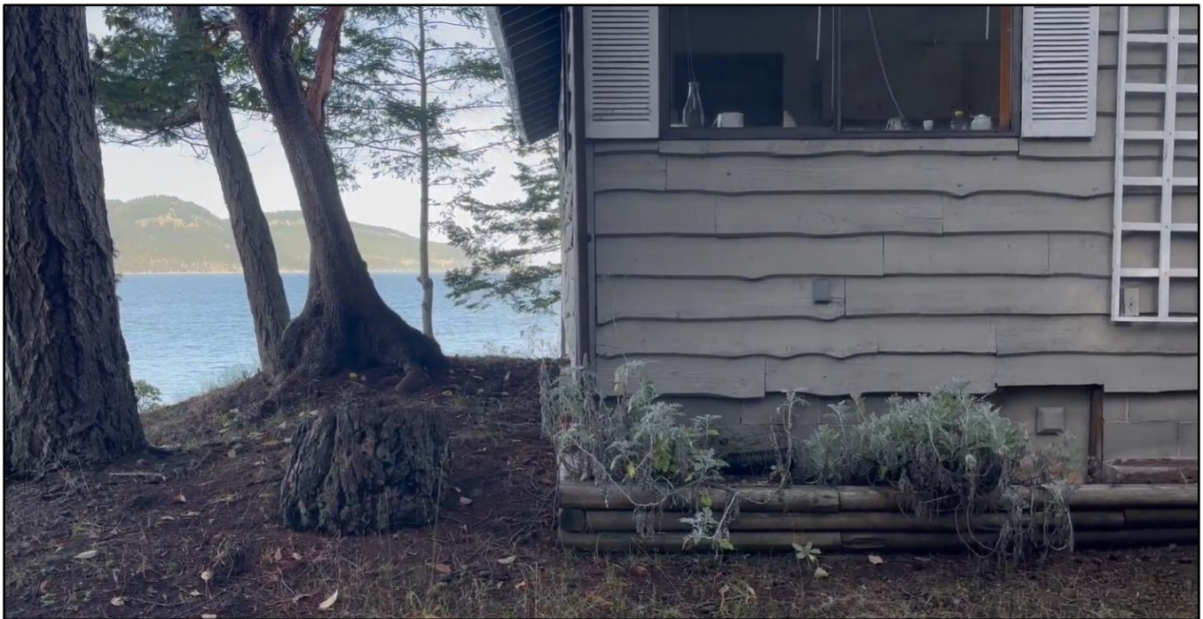
NORTH-WEST CORNER OF EXISTING DWELLING, LOOKING EAST
