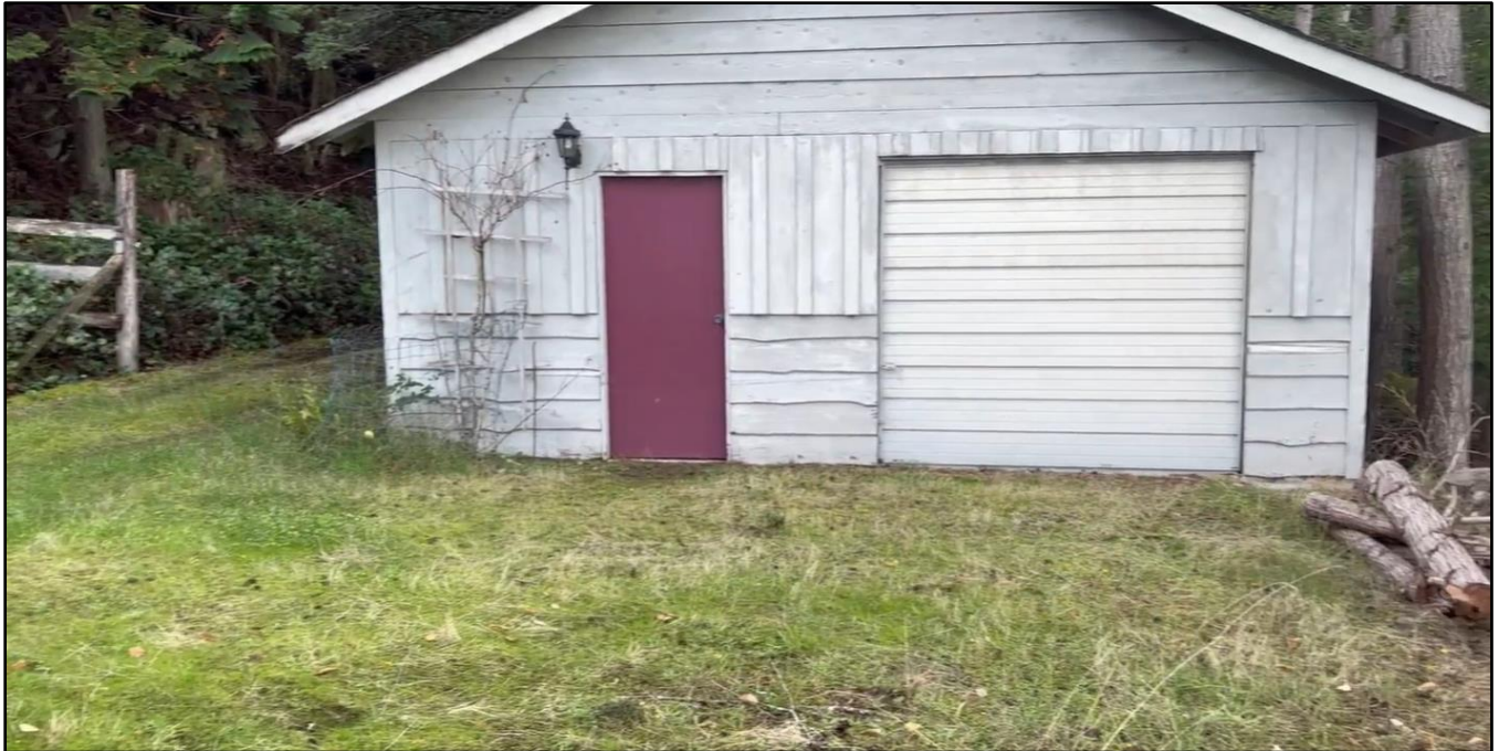
EXISTING GARAGE, LOOKING WEST
