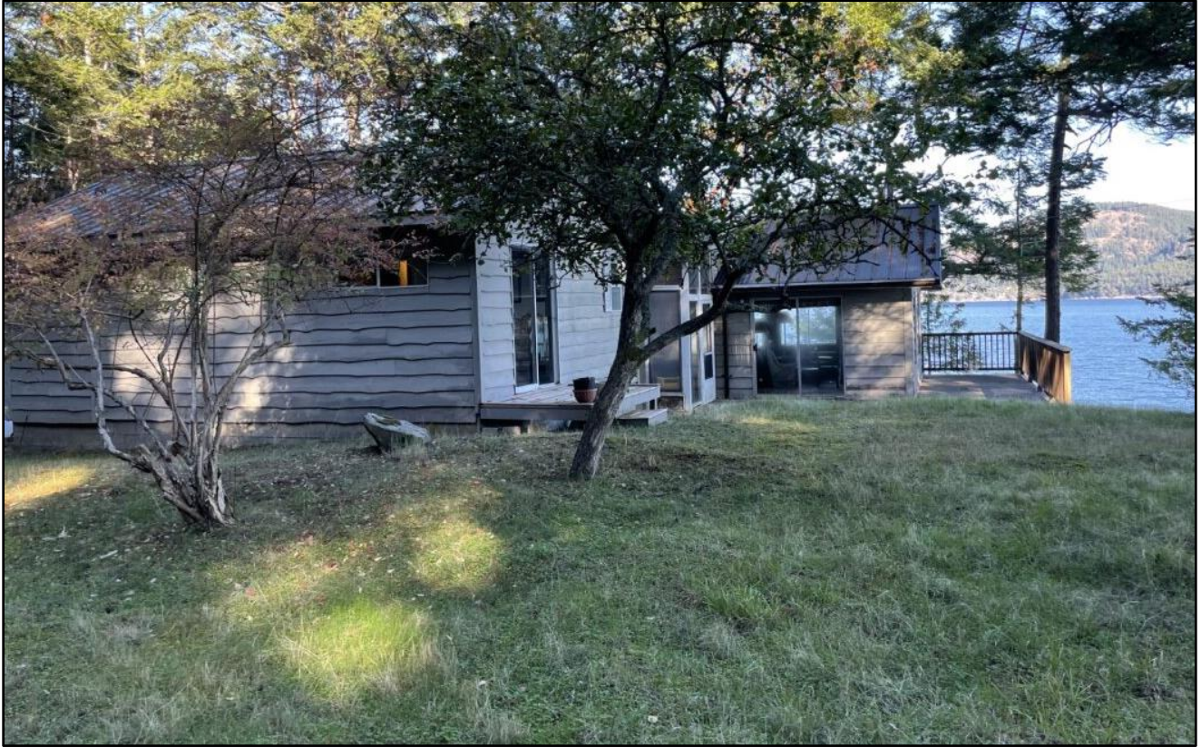
EXISTING DWELLING AND DECK TO BE REMOVED, LOOKING NORTH-WEST
