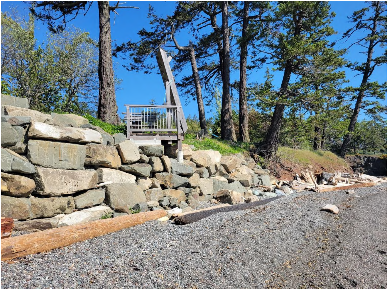
SHORELINE WALL AND STAIRS, LOOKING NORTH-WEST
