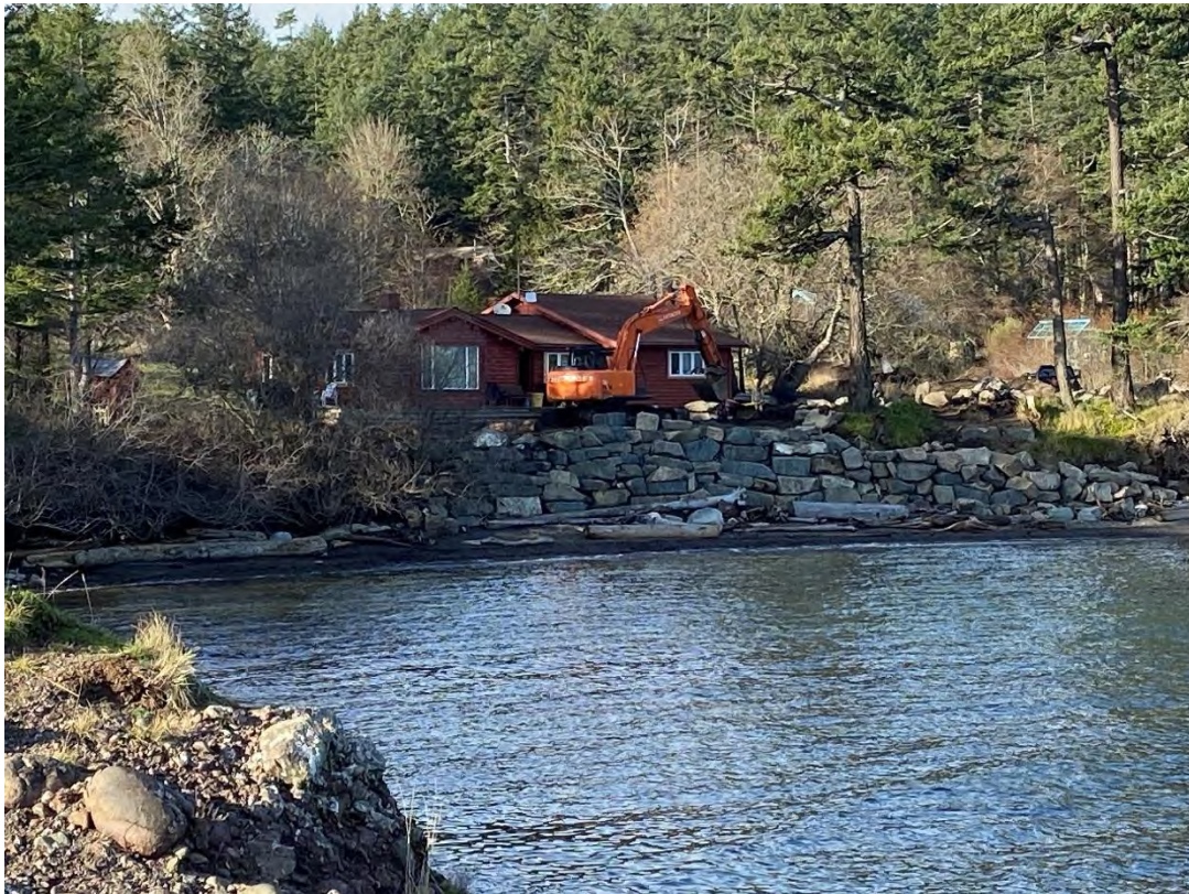
SHORELINE WALL UNDER CONSTRUCTION, DECEMBER 12 TH 2023, LOOKING WEST
