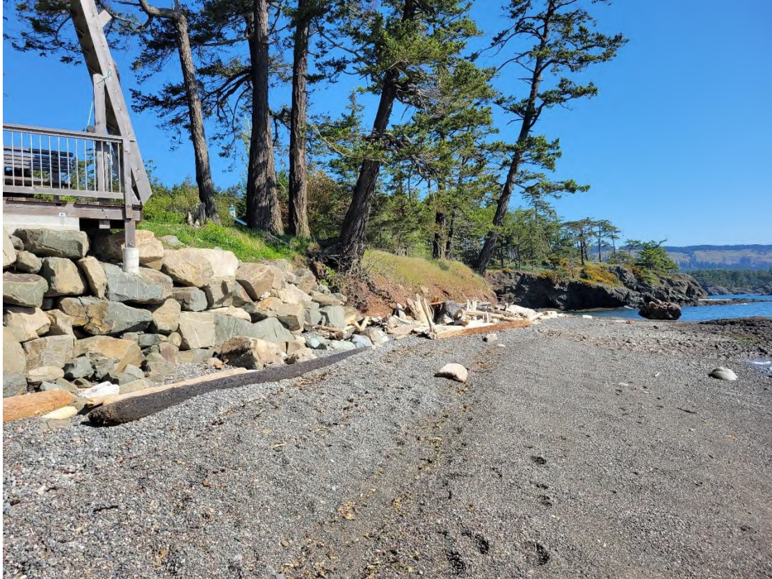
SHORELINE WALL AND STAIRS, LOOKING NORTH UP GOWLLAND POINT BEACH
