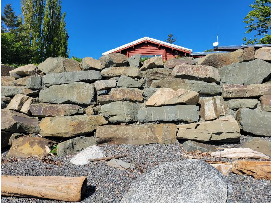
SHORELINE WALL LOOKING WEST
