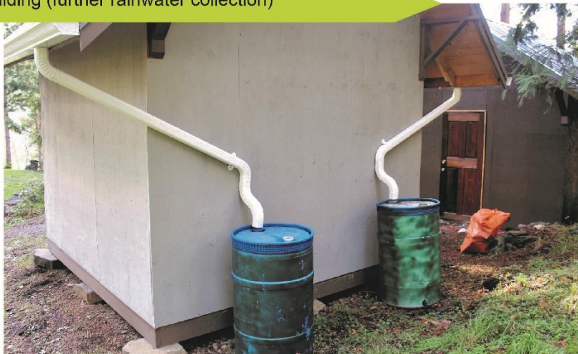
Five: Rear of accessory building (further rainwater collection)
