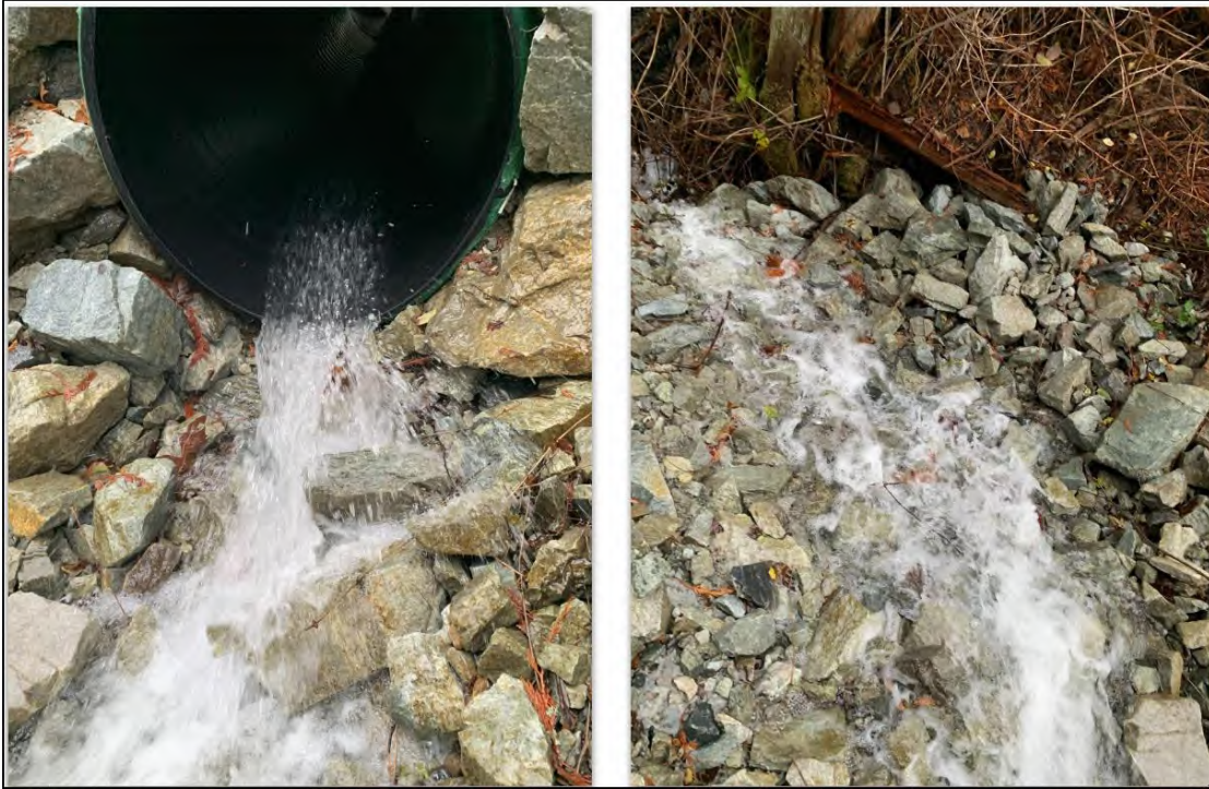
FIGURE 4: DOWNSTREAM VIEW OF COMPLETED INSTALLATION OF CULVERT WITH WATER FLOWING
