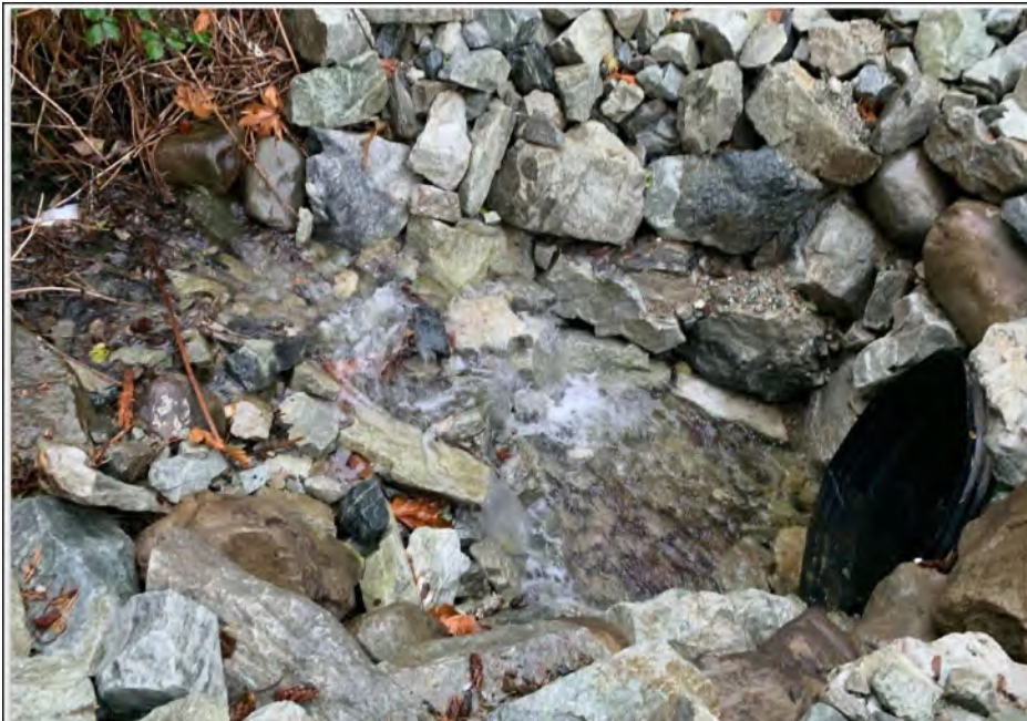
FIGURE 3: UPSTREAM VIEW OF COMPLETED INSTALLATION OF CULVERT WITH WATER FLOWING
