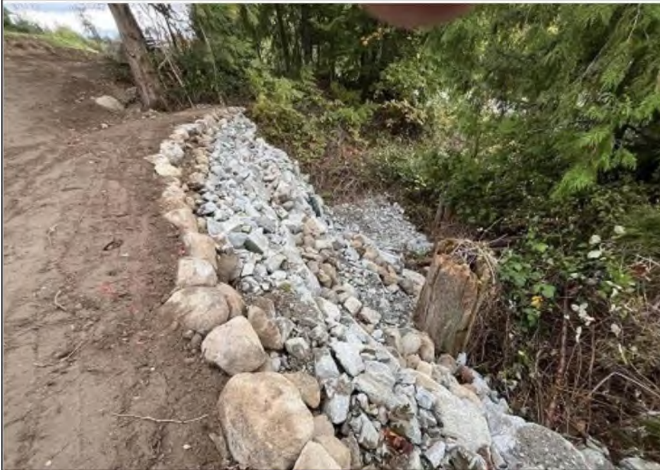
FIGURE 2: DOWNSTREAM VIEW OF COMPLETED INSTALLATION OF CULVERT
