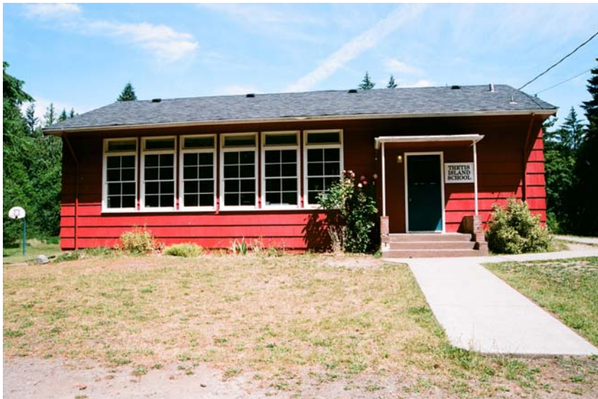
Thetis Island School - Photo by Brett Korteling
