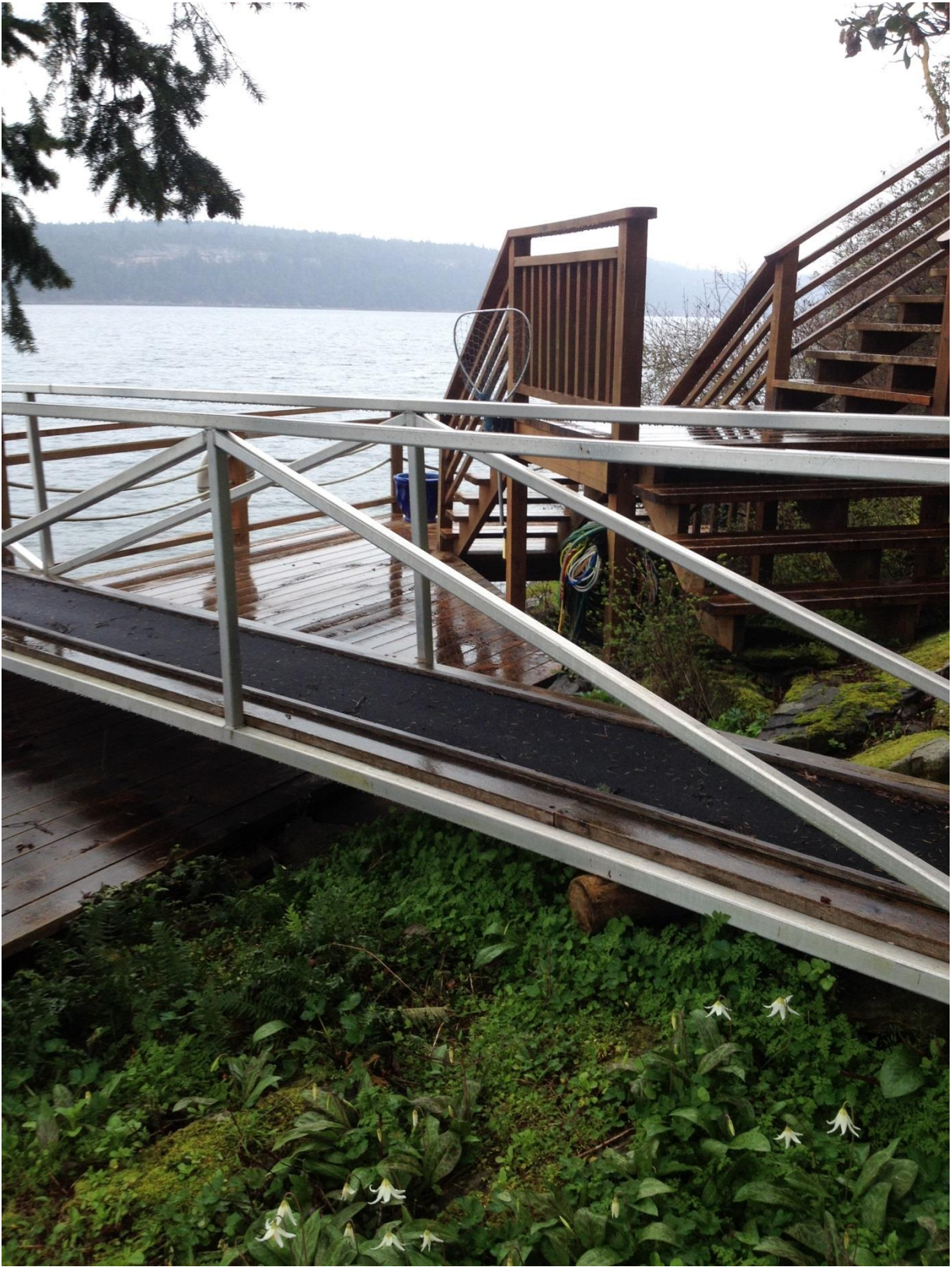
Photo 9: Access stairs connecting to “Waterfront Walk” structure
