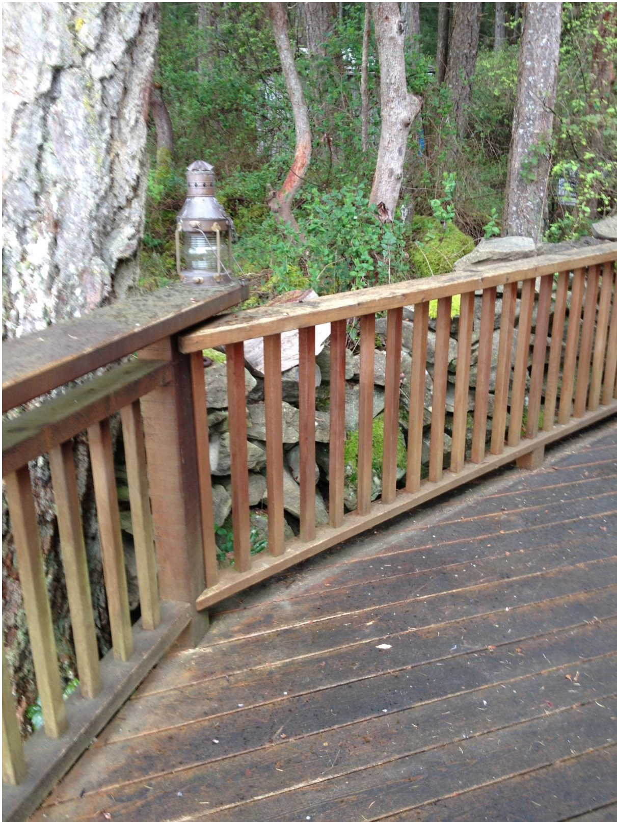
Photo 1 : View of Patio, facing south
