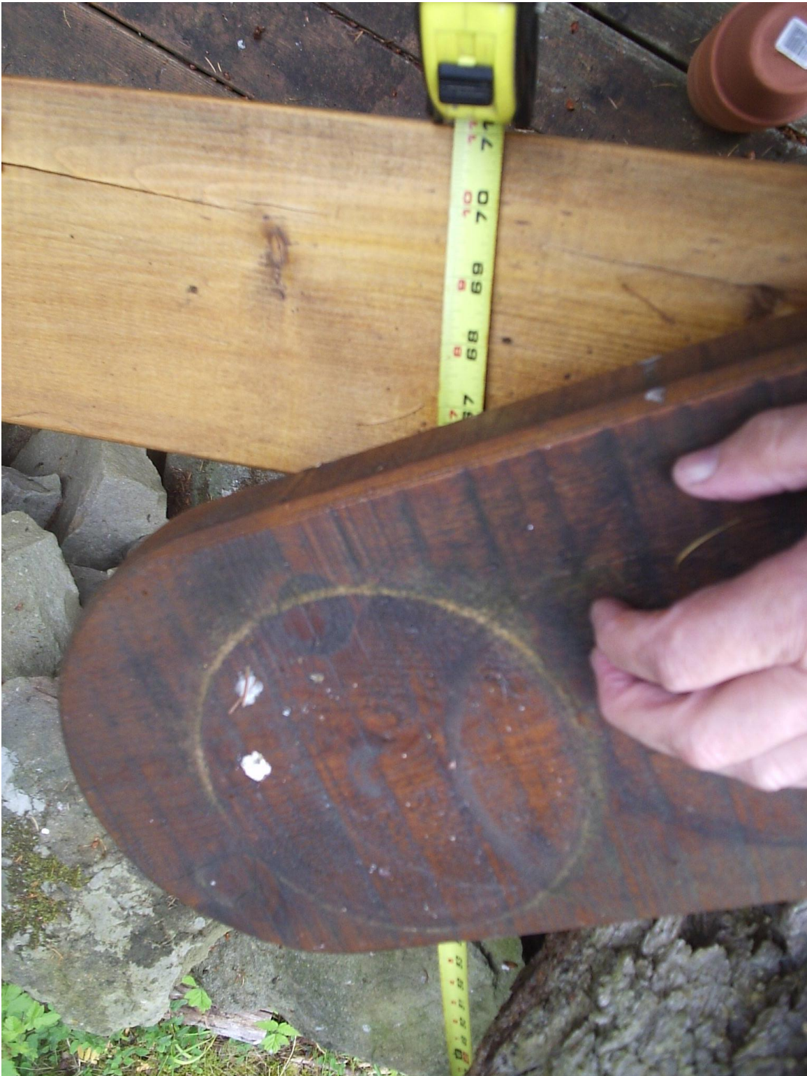
Photo 5: Distance of about 66 inches (5.5 feet / 1.67m) from southeast property line to inside of patio railing
