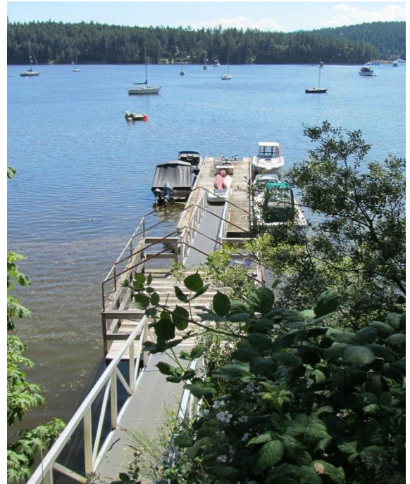
Photo 8: Overwater Structures (Dock) Credit: K. Nichols
