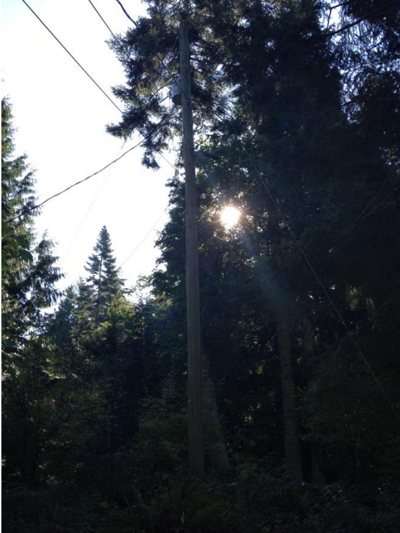
Figure 9: Existing Hydro pole to south of proposed building site (facing south)
