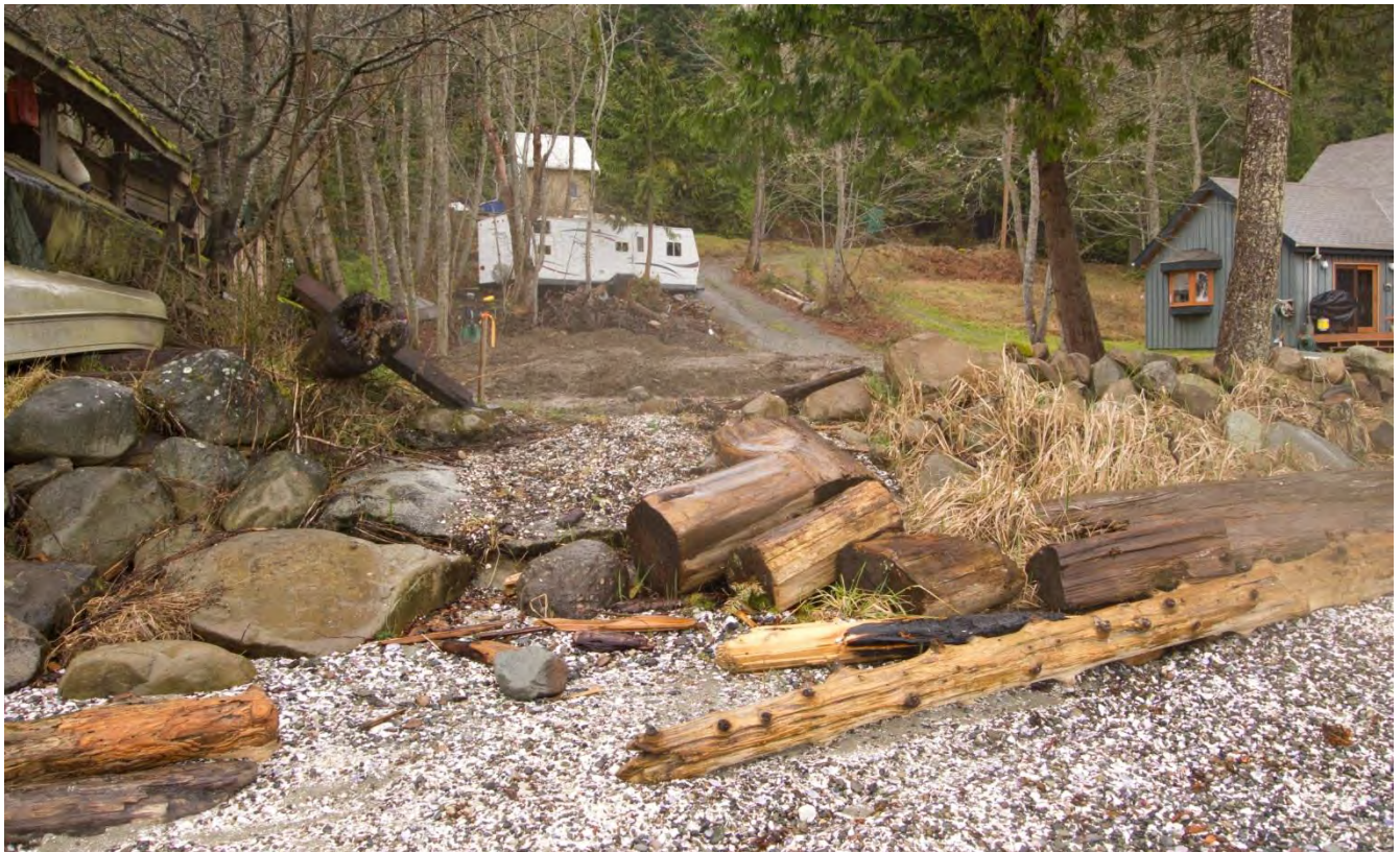
LOT 137 is being developed. Boulders and logs have been placed at the shoreline.
