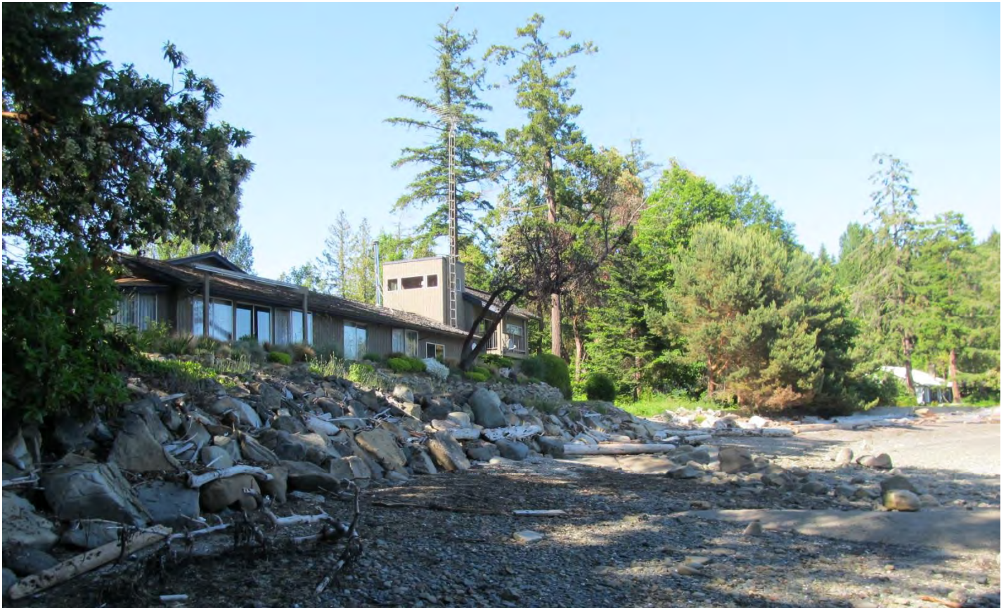
The rip rap wall facing east to the rest of the beach.
