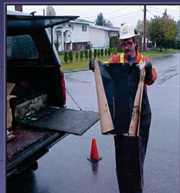
Field-Made Pole Bandage
