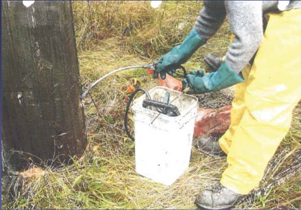
Fumigant placed into drill holes using hand-operated sprayer
