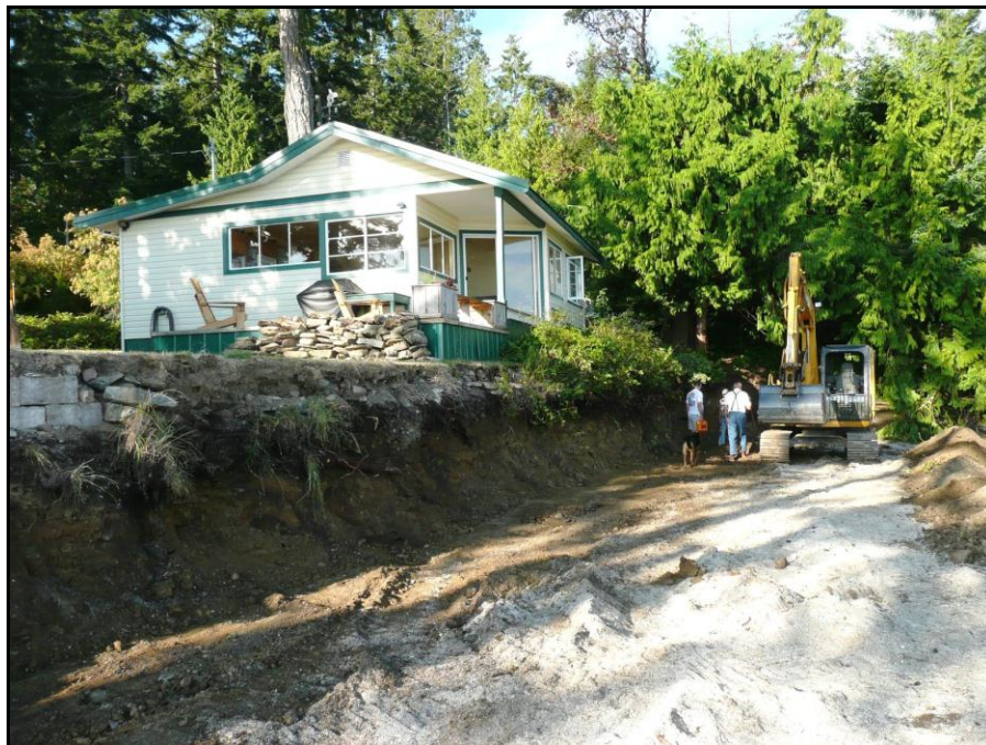
Figure 1 Sheering and leveling of bank
