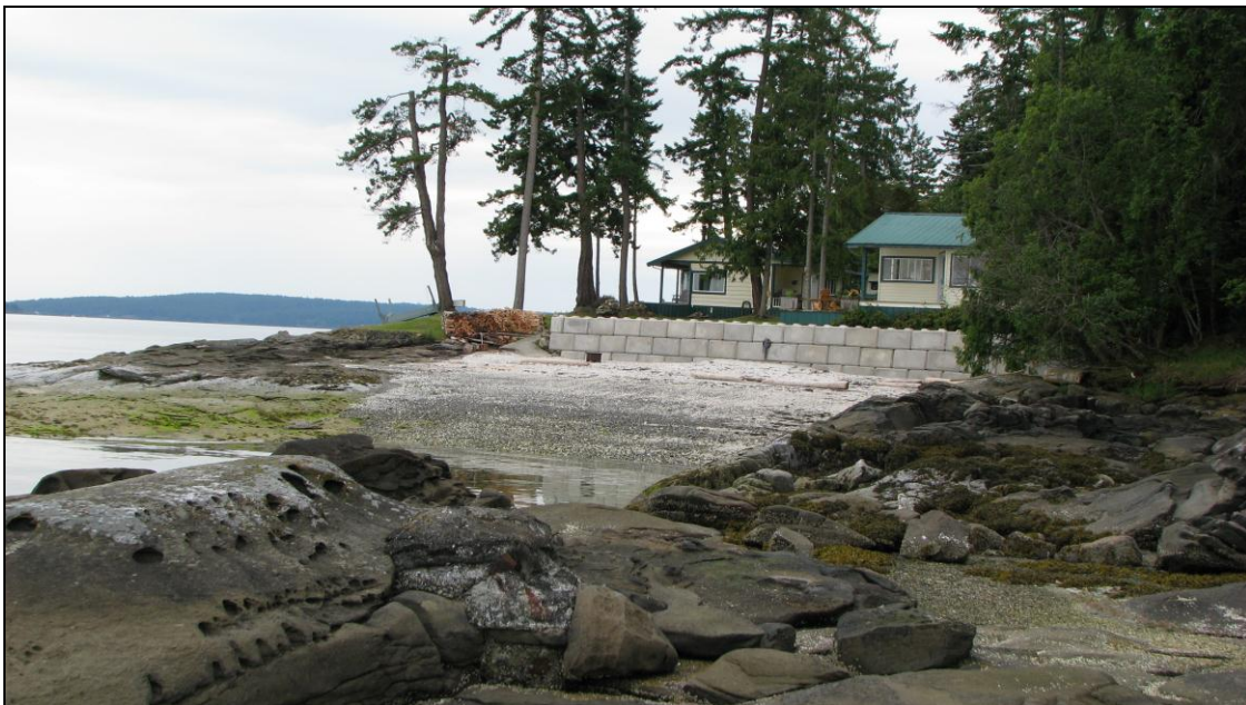
Figure 3 Finished seawall showing shell beach
