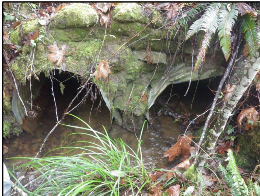
Photo 6. The outlets of the CMPs that convey Ralston Creek under Lakeview Road. These two CMPs are embedded and passable by fish.
