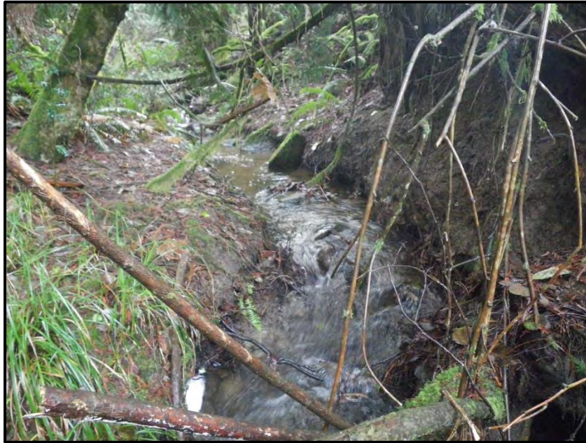
Photo 7. Looking upstream at Ralston Creek from the inlet of the two CMPs that are positioned under Lakeview Road.
