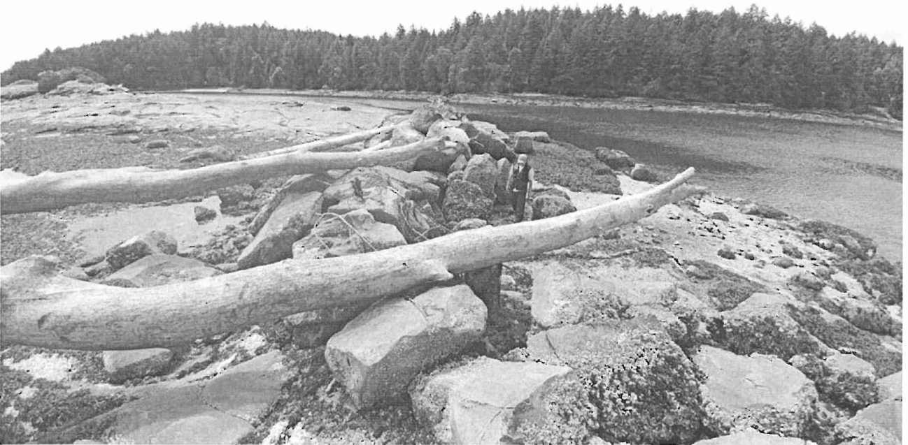
Figure 3 Photograph of existing breakwater constructed of large sandstone boulders atop of sandstone bedrock intertidal reef south of Kendrick Island. Gary Drouillard, Lyackson First Nation, in centre. Looking south, June 9 th , 2017.
