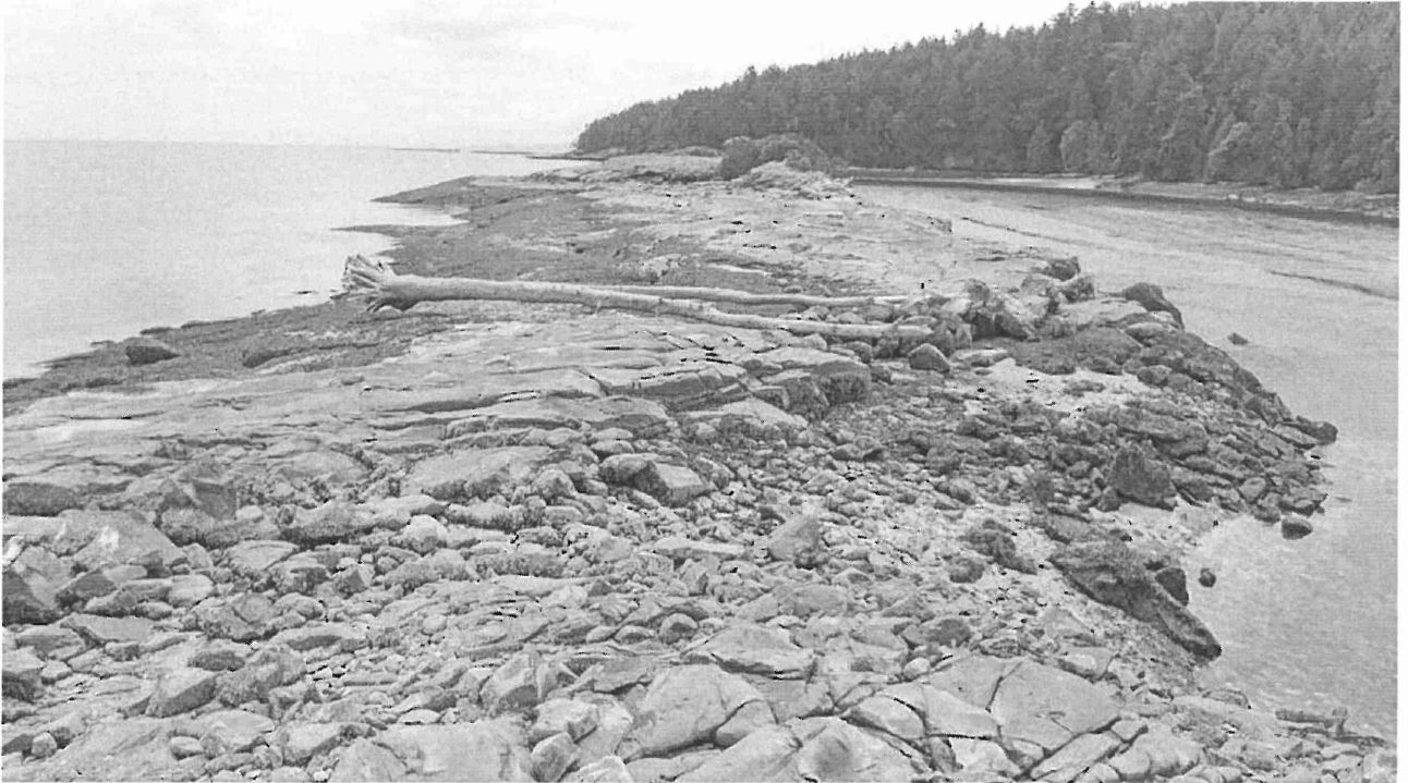
Figure 2 Photograph of Proposed Breakwater Improvement Area, Kendrick Island, Existing breakwater is located to right of centre of photograph where two large driftwood logs have been caught among the boulders, which protect the dock and mooring buoys from storms, wave action, high tides and floating debris. Looking southeast, June 9 th , 2017.
