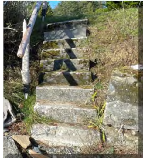
Photo #2 - on the right is the stairs of the same concrete seawall/hard armour. Photo credit D. Fenton, Oct 26, 2023.
